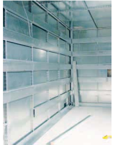
Substructure for the installation of ferrite absorbers
